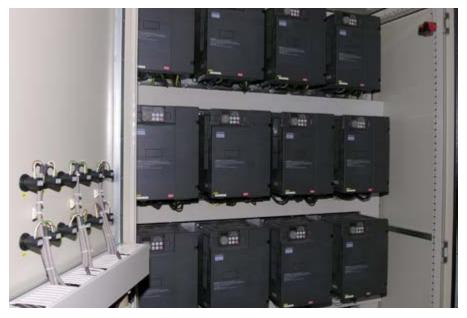
Inverters mounted in an electrical cabinet
