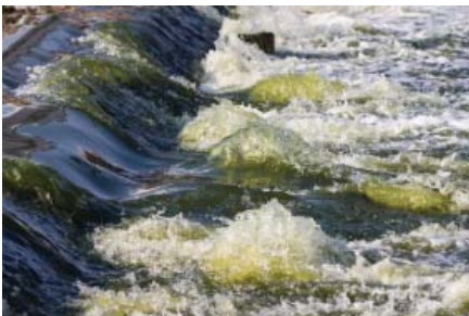
Weir control system
