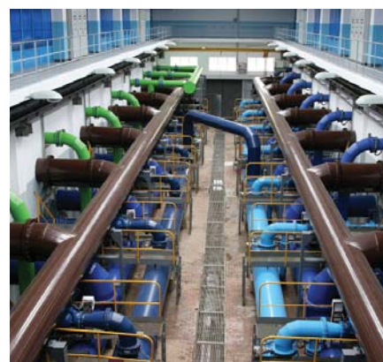
Modern water plant control systems built around Mitsubishi Electric control systems can help water companies reduce energy costs and boost operational efficiencies.
