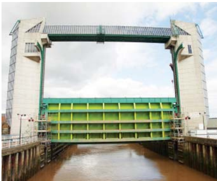
Flood control system
