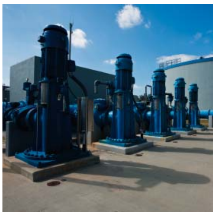
Powerful centrifugal pumps and other pump types are used to protect against flooding.
