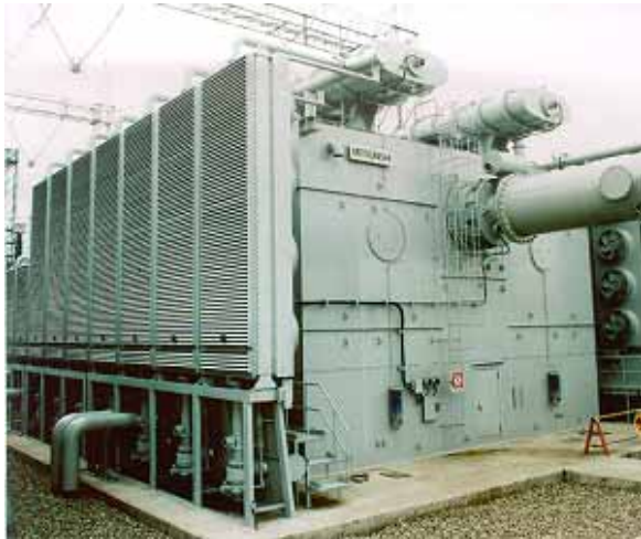
Fig. 5 The 1,000kV transformer installed on site.
