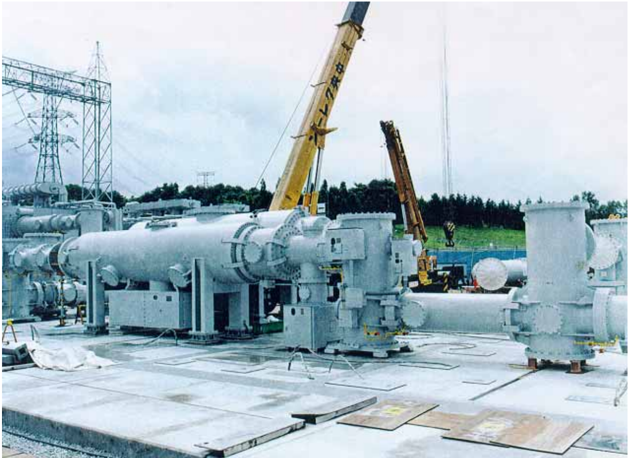
Fig. 2 A photograph of 1,000kV GIS installation.
