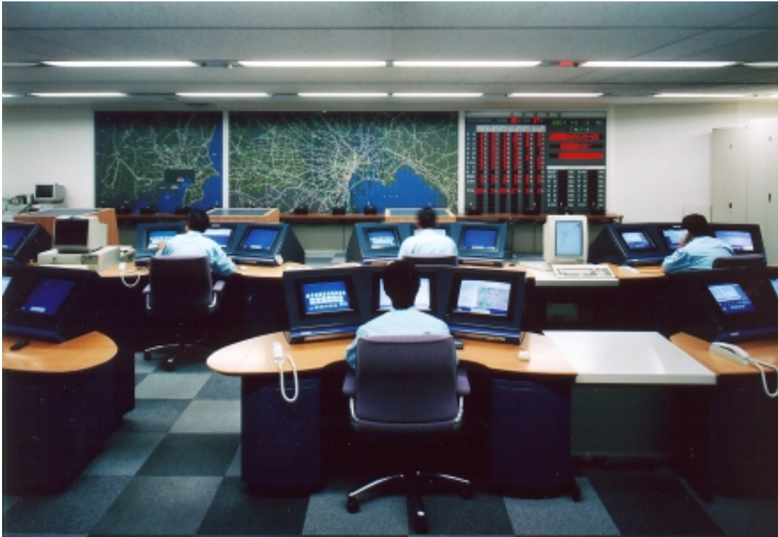
Fig. 2 A photograph of the monitoring center.
