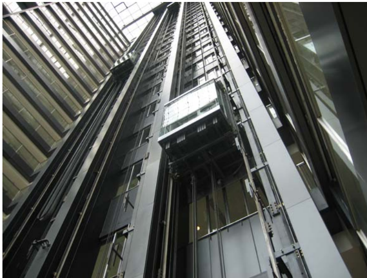
Photo 4 Observation cab running inside void area
