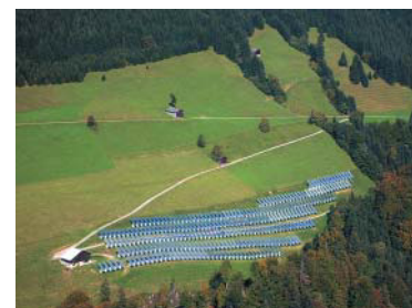
Fig. 4 Installation sample of small-scale power generation
